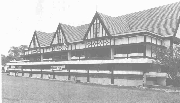
Selangor Club, established in 1884 to meet the social and recreational needs
